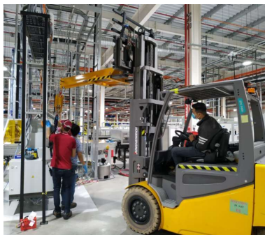
Figure 7. Replace the roller using forklift
